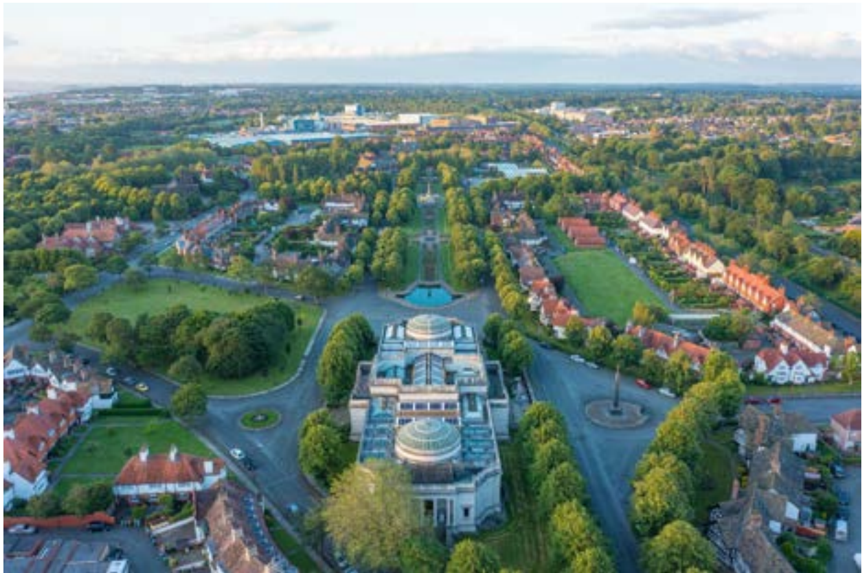
Figure 1: Aerial view of Port Sunlight, 2021. View looking south from the Lady Lever Art Gallery towards the Unilever campus. View shows the axial, City Beautiful-inspired village centre, the generous landscapes, superblock layout, monuments and setting. Photograph courtesy of Stratus Imagery Ltd.
