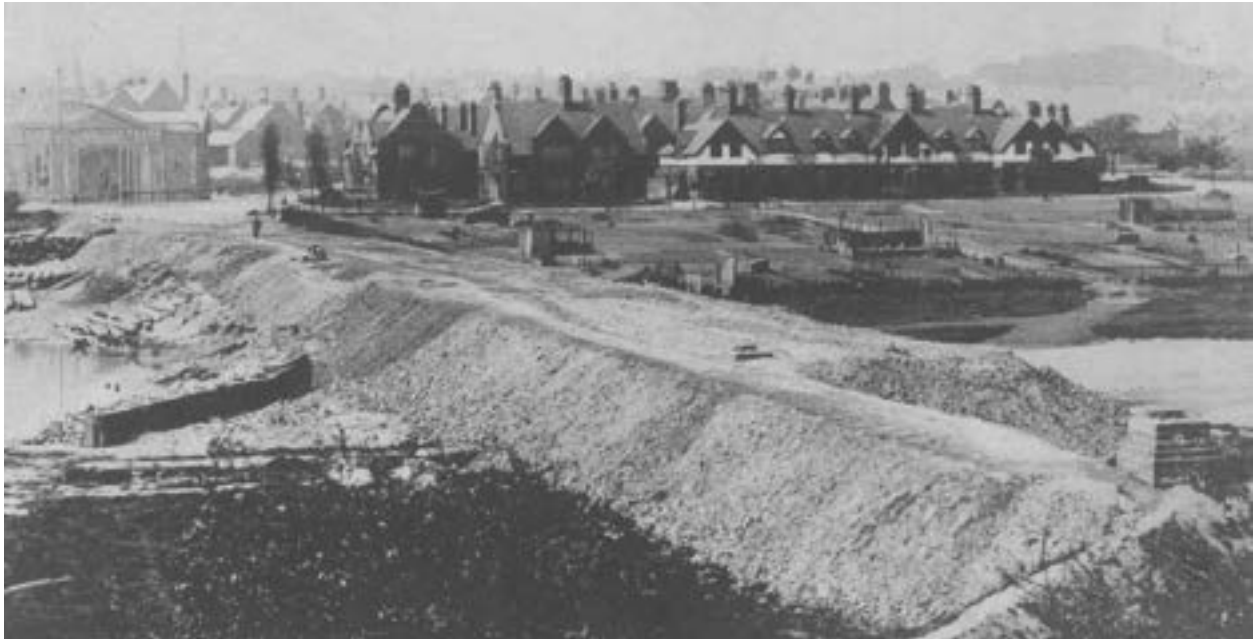
Image 2: Tidal creeks covered 25 acres of the Port Sunlight estate. By 1901, Lever Brothers started work to dam and divert the waterways that crossed the estate. This work took nearly nine years for the company to complete and enabled the introduction of a City Beautiful-inspired site plan at the village centre. This view shows the dam under construction c1903. Victoria Bridge became redundant during this work and was buried. Reproduced by kind permission of Unilever PLC from an original in Unilever Archives.
