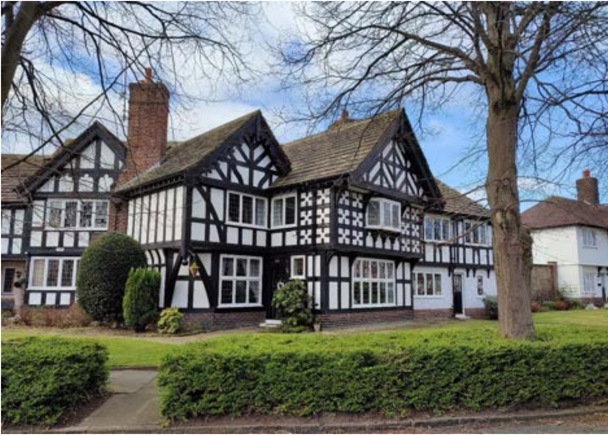
Image 5: Detail view of the subsidised inter-war housing developed by Lever Brothers (designed by James Lomax Simpson, 1924) to introduce axial site planning and vistas both to and from the Lady Lever Art Gallery. This housing replaced earlier terrace blocks and a street plan developed by Lever Brothers. Photograph by Heather Alcock, 2022.
