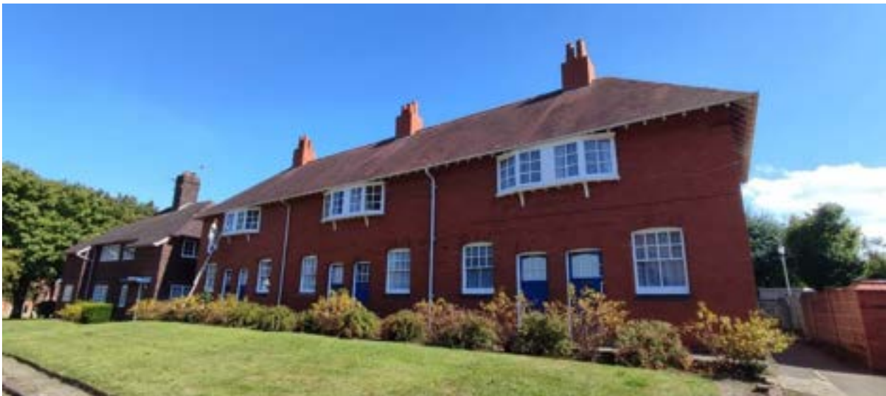
Image 14: View of 8-12 Bolton Road, which was converted from six, small terrace houses into three larger cottages in the 1970s. Photograph by Heather Alcock, 2022.
