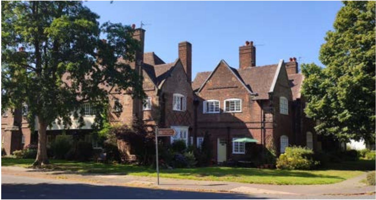
Image 11: 13-17 The Causeway/47-50 Queen Mary's Drive (James Lomax Simpson, 1913) were converted from single family homes into flats in the 1970s. The development was sensitively refurbished in the 1990s (See Image 12) with no alterations to the primary or secondary facades. Photograph by Heather Alcock, 2022.
