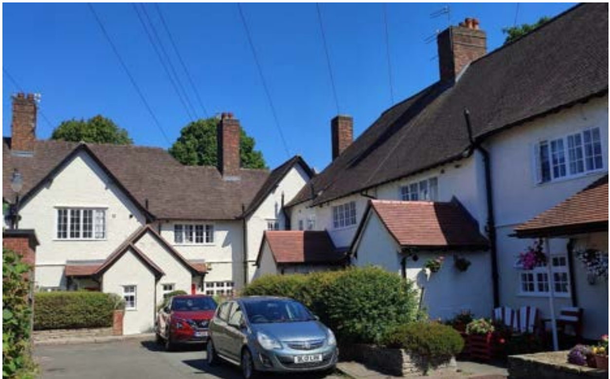
Image 12: View of the backs of social housing flats at 13-17 The Causeway/47-50 Queen Mary's Drive. These improvements, including small extensions, were introduced in the 1990s. These improvements are sensitively designed and concealed from public view. Photograph by Heather Alcock, 2022.
