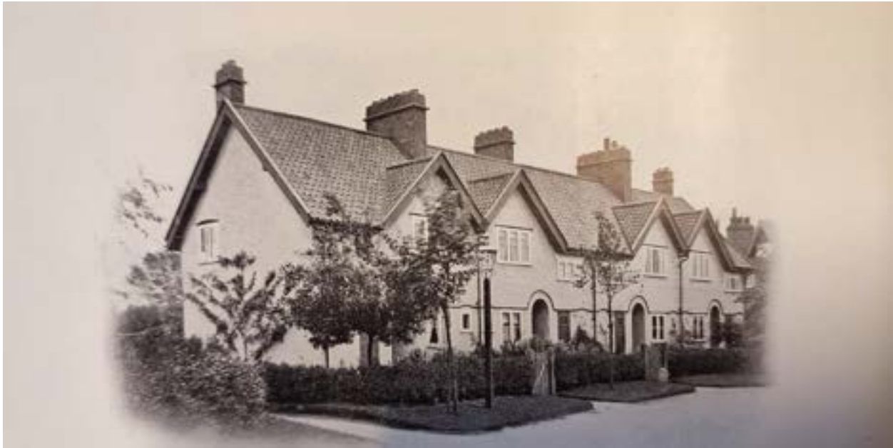
Figure 10: Example of housing at New Earswick. Identified as 'Type II', this block of housing had four separate residences. The lounge extended from the front to the back of the houses with a scullery to the side of the lounge opening to the back of the property. Although practical, this type of house was not popular with tenants and its design was modified to suit their preferences. From "New Earswick, York" by the Joseph Rowntree Village Trust (1913), p16. held in the JRVT Collection at the Borthwick Institute, University of York, reference NE 21/15.
